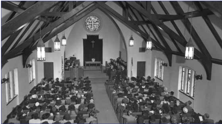
Sanctuary before Lattner Organ Installed
